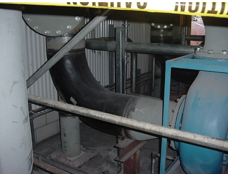
FIGURE 4. This elbow is shown with an insertion panel tab conditioner to pump connection. (Source: Fluid Components International)
