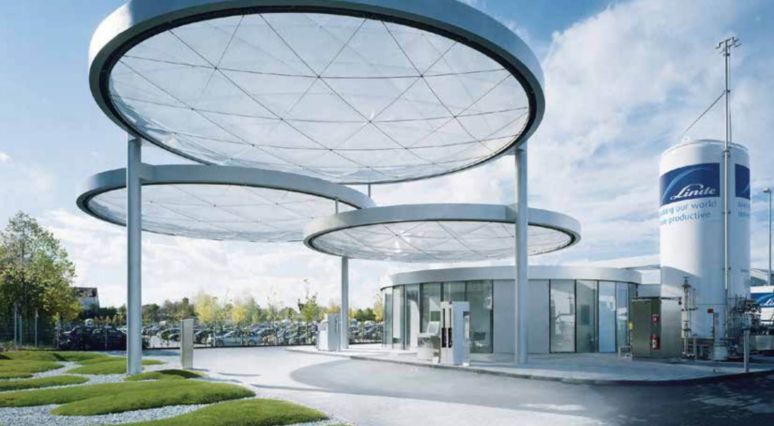
(Left) Linde hydrogen refinery in Texas; (above) Linde's hydrogen center in Unterschleissheim, Germany.
