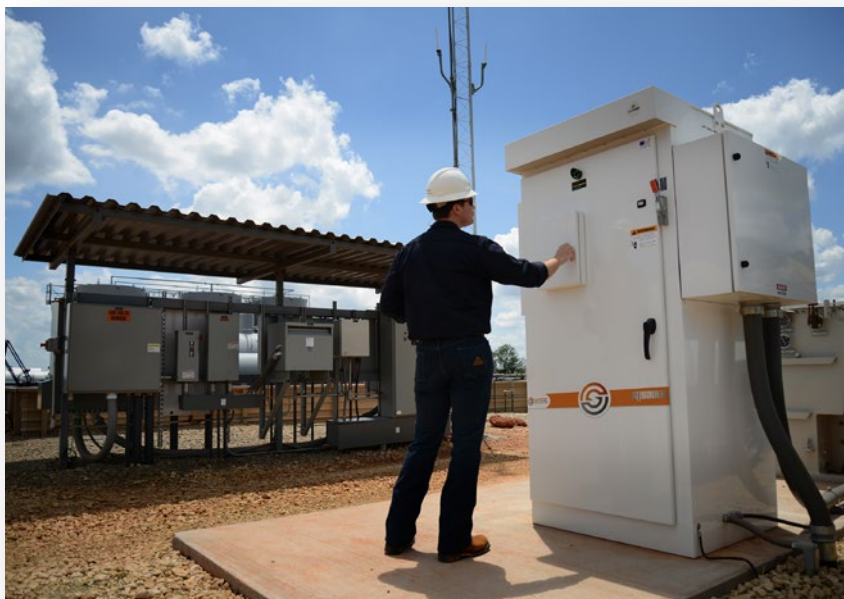
A pumper checks electric submersible pumps and well conditions in West Texas. (Source: SPOC Automation)
