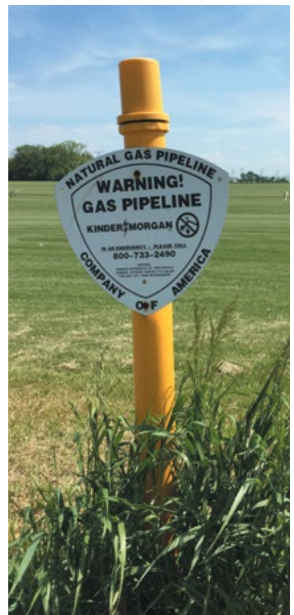
This route marker guards a Natural Gas Pipeline of America right-of-way in Illinois. Source: Kinder Morgan Inc.
