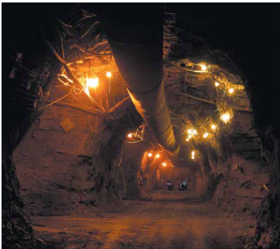
WSP USA has constructed more than 80 hard rock caverns in the U.S. to store propane or butane. Source: WSP USA
