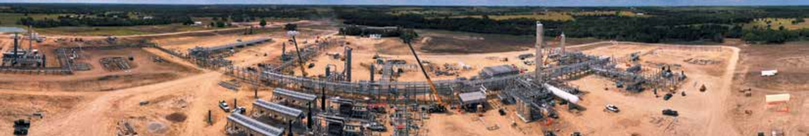
The Battle Horse processing plant, with a capacity of 200 million cubic feet per day, will be the hub of Aspen Midstream's new South Texas system. Source: Aspen Midstream LLC
