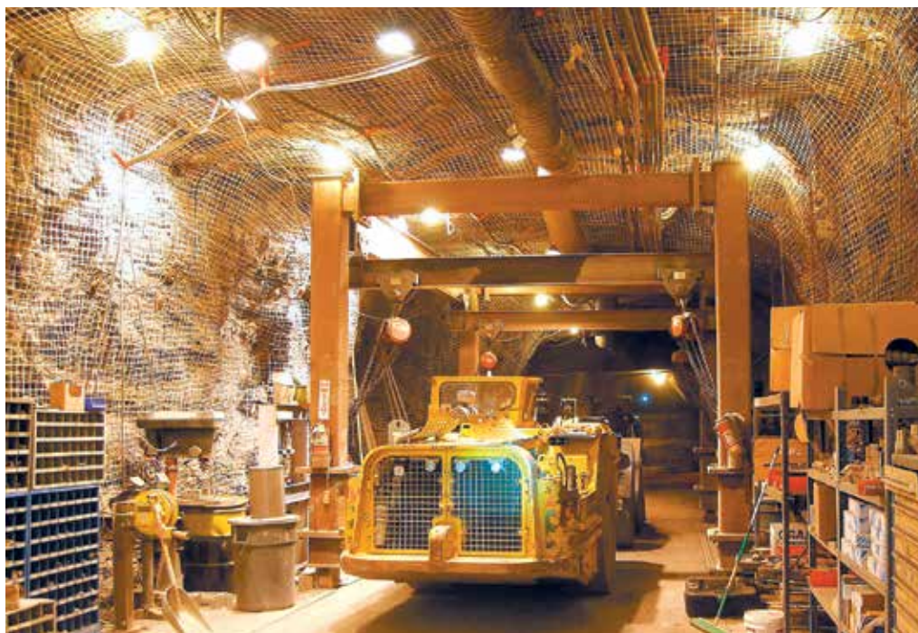
When a mined area is large enough to lower drilling and hauling machines into place, items are dismantled, lowered down the production shaft and assembled at mine depth. Source: WSP USA
