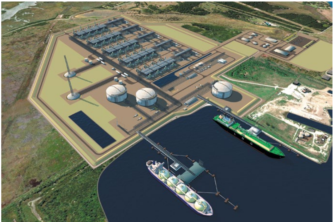
Tellurian Inc. says its Driftwood project outside Lake Charles, La., will be among the lowest-cost LNG liquefaction operations. First production could come as soon as 2023. Source: Tellurian Inc.
