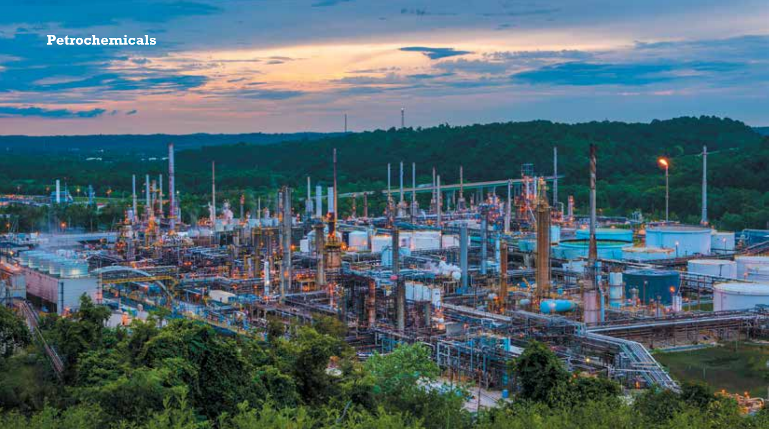
Processing and refining along the banks of the Ohio is nothing new. Marathon Petroleum's Catlettsburg, Ky., refinery—where Kentucky, Ohio and West Virginia come together—began operation in 1916. Source: Marathon Petroleum
