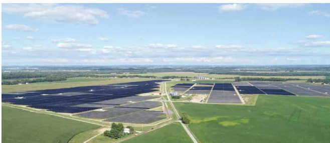
National Grid Renewables
