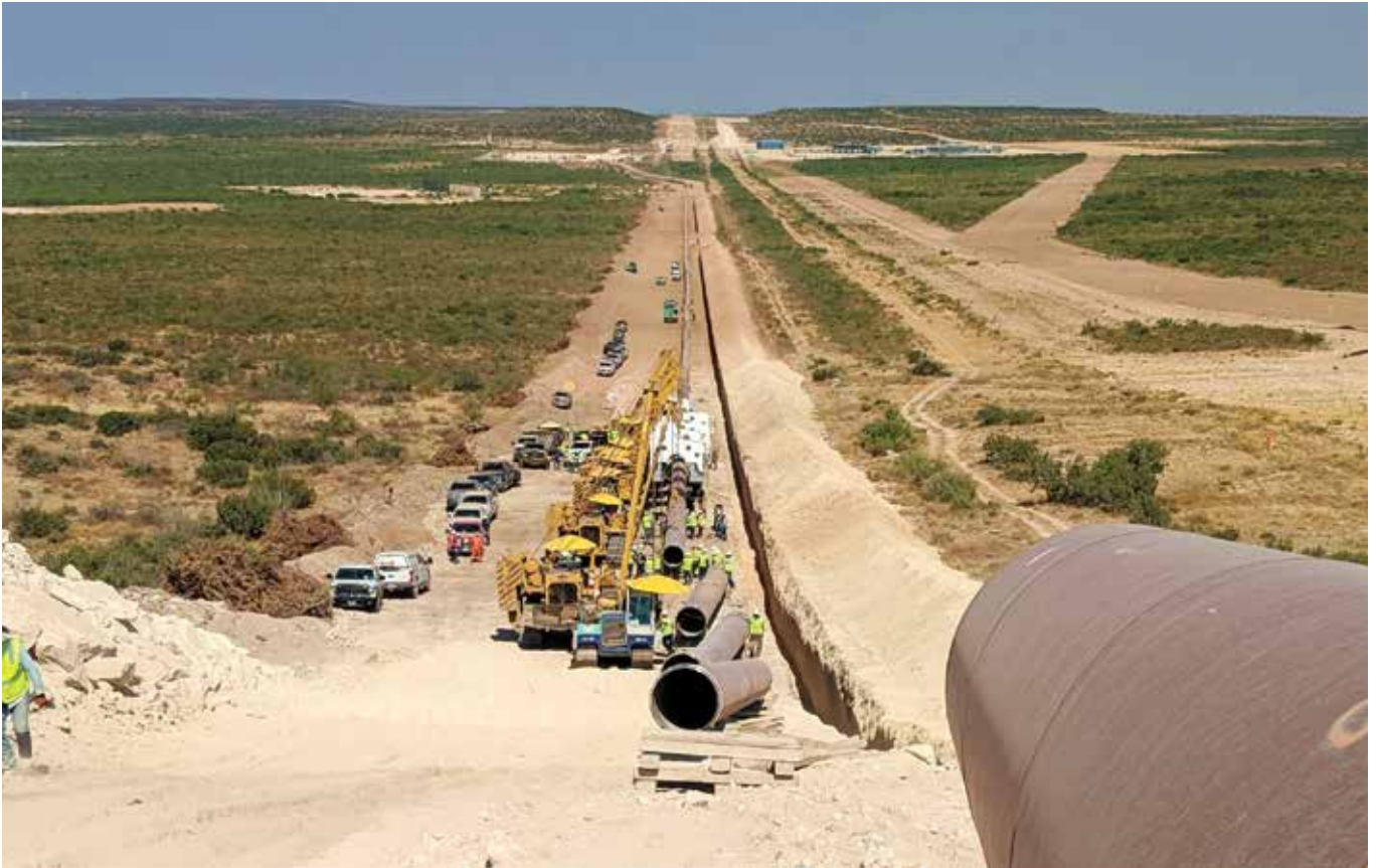
The Whistler natural gas pipeline, seen under construction, transports natural gas from the Permian Basin. Its expansion, completed in September, increased its capacity to 2.5 Bcf/ from 2 Bcf/d.
