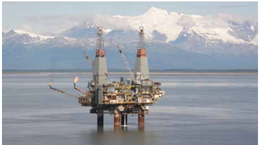
Hilcorp Trading Bay Platform in Alaska
