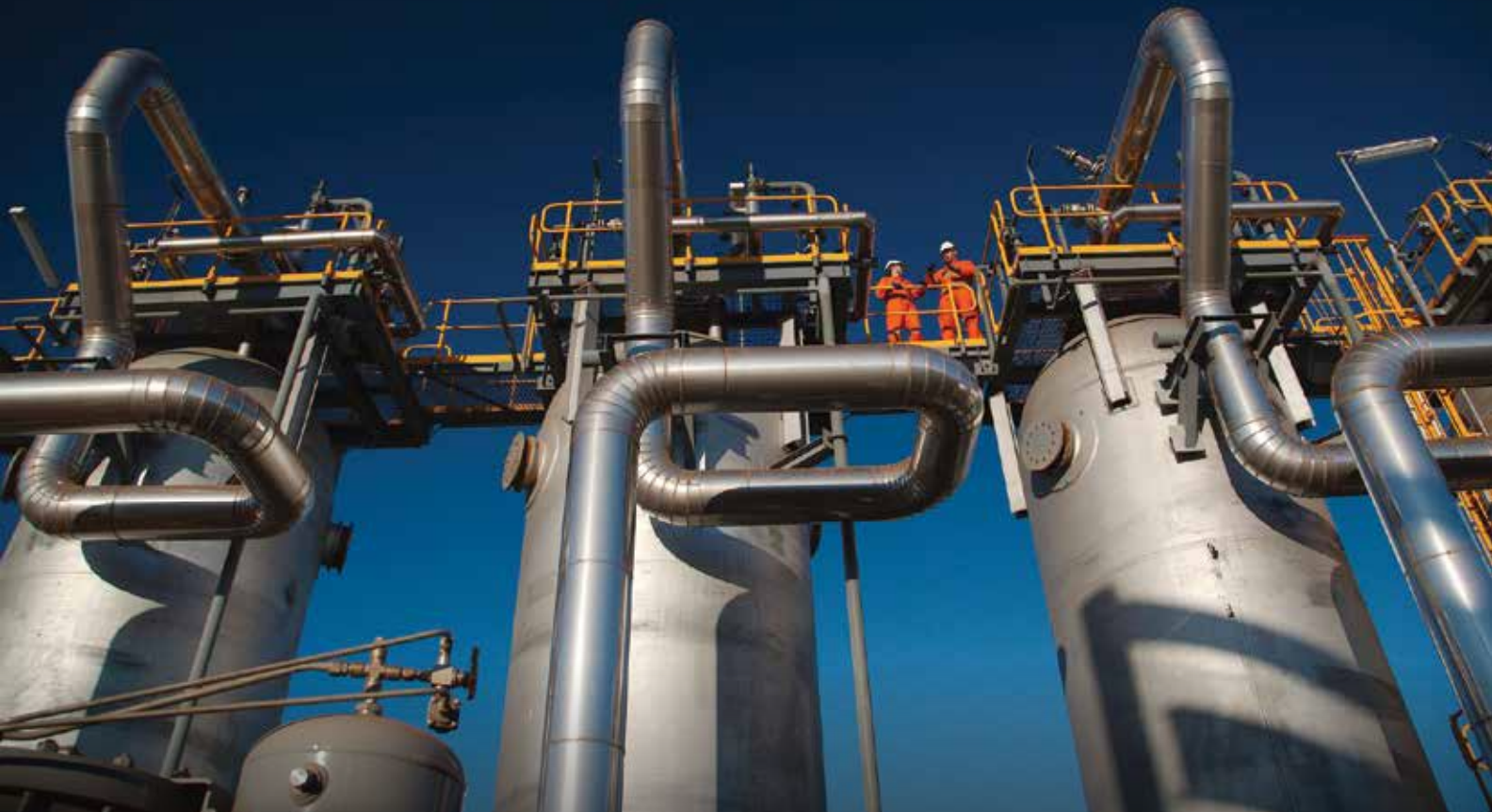
Macedon offshore gas field in Onslow, Western Australia.
