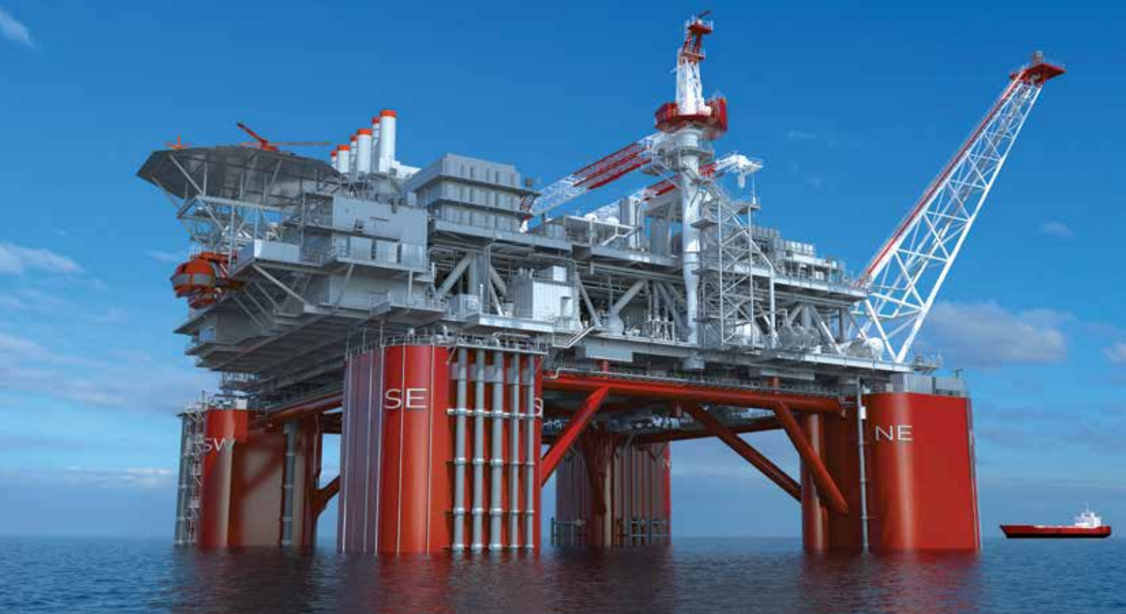
Rendering of planned FPU for the deepwater Trion project in the GoM.
