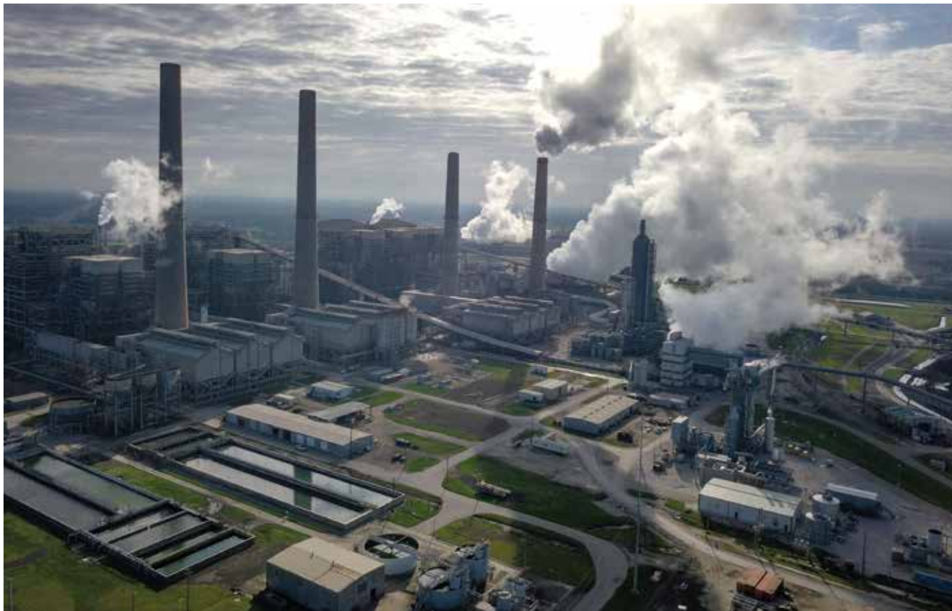
Aerial photo of W.A. Parish Generating Station in Fort Bend County, Texas. Petra Nova was designed as a post-combustion carbon capture treatment system to reduce atmospheric exhaust emissions from the power plant.
