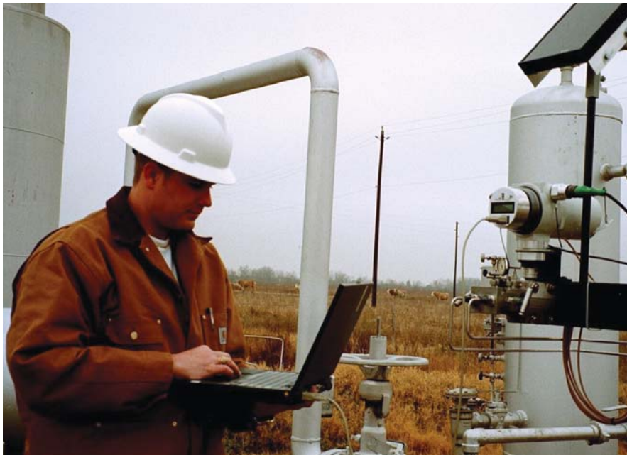
Programming the Smart-Alek unit to collect and send gas flow data over wireless communication networks.
