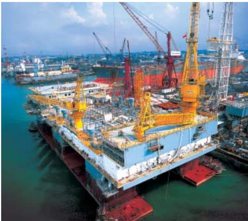
Singapore hosts a world-class marine construction industry.
