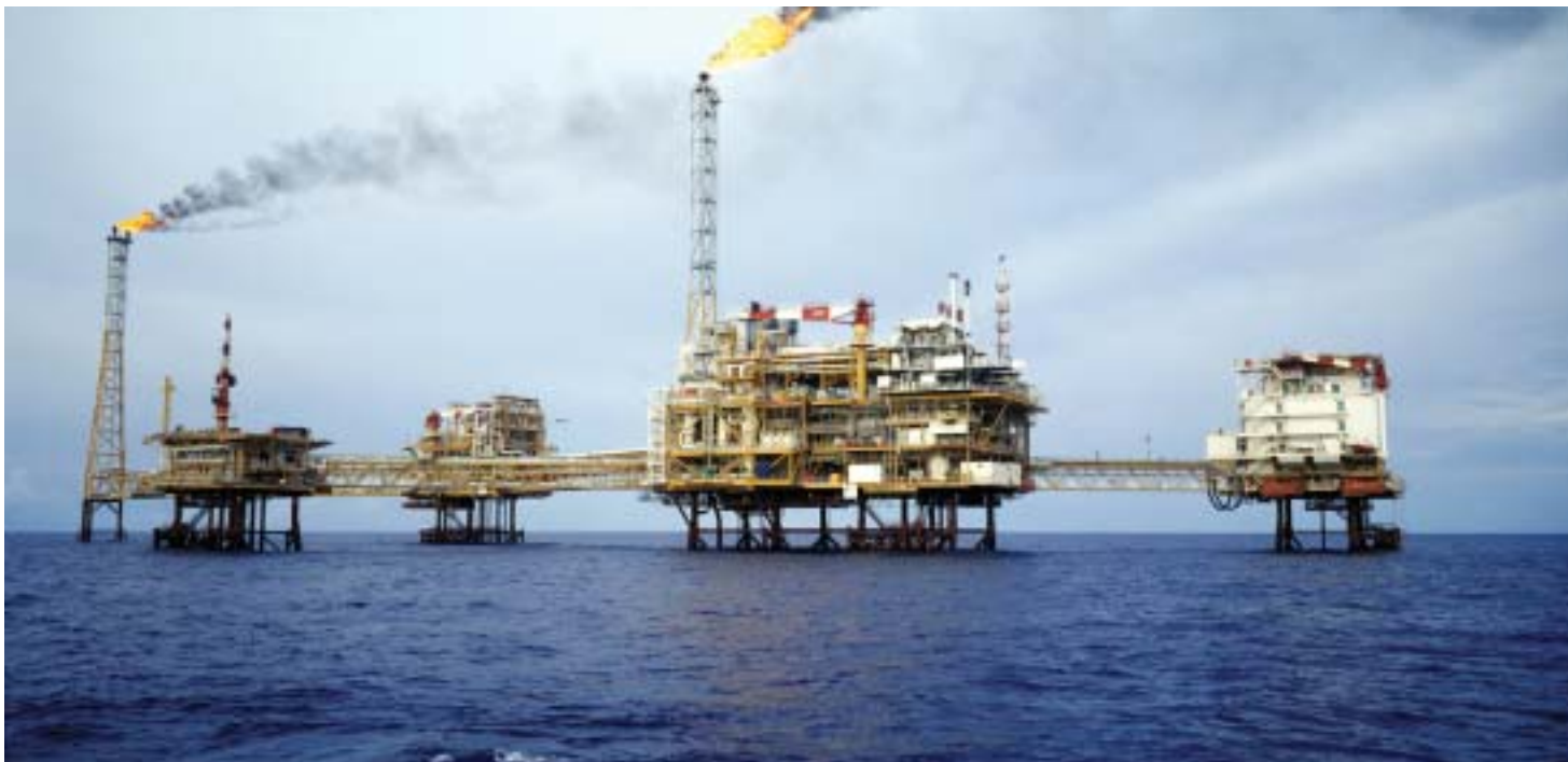
The Bongkot gas field production facilities in the Gulf of Thailand.
