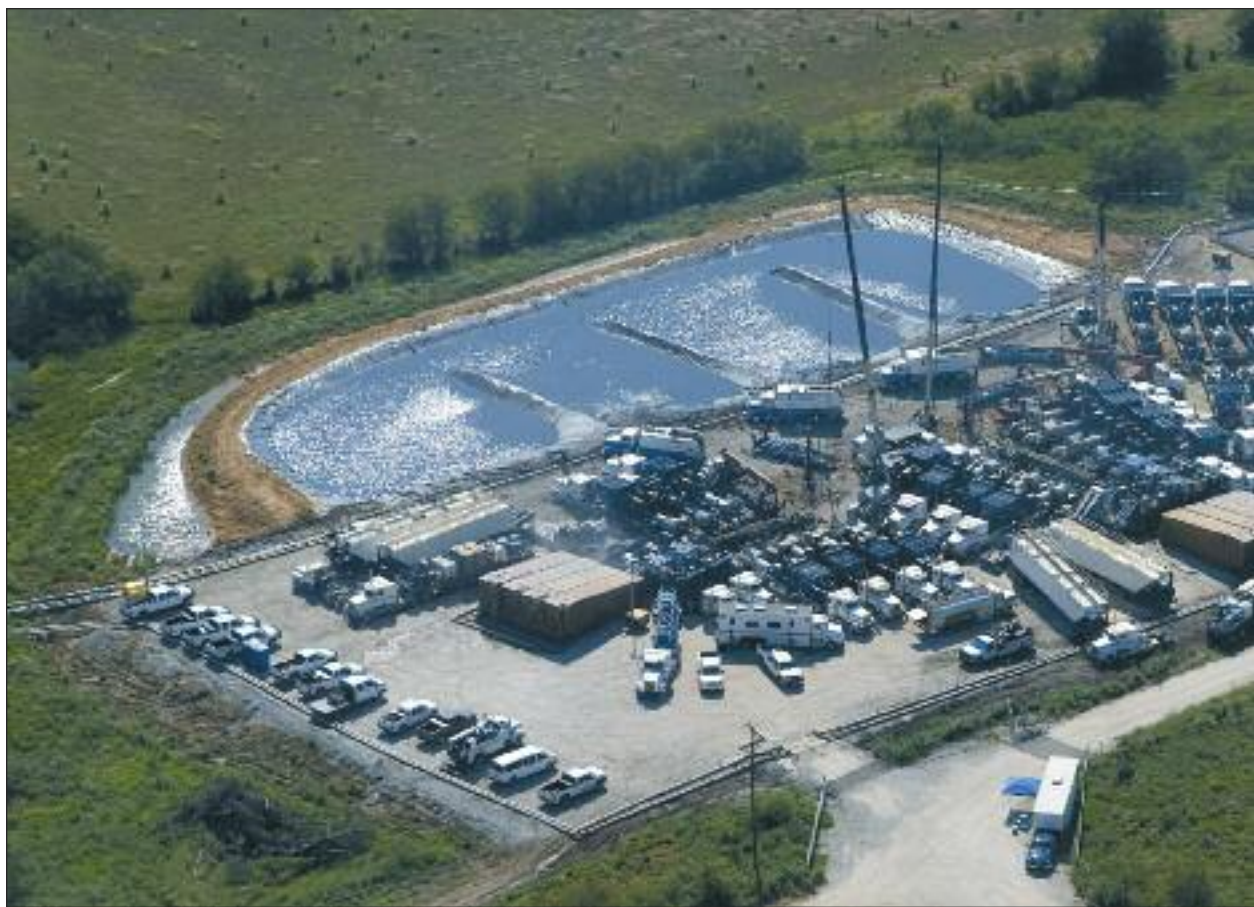
A BJ Services frac spread operates beside carefully hoarded frac water, which is exceedingly scarce despite the green appearance of the land. Photo courtesy of BJ Services
