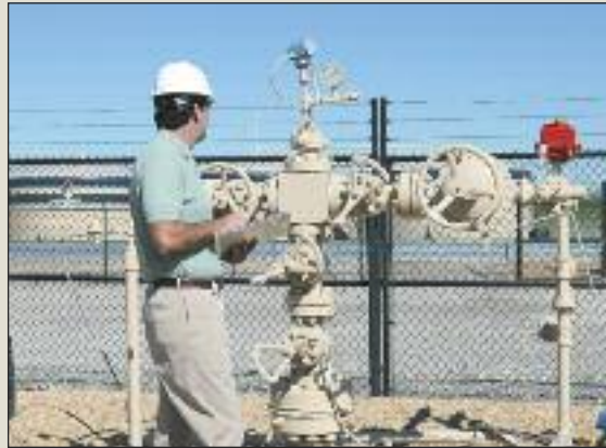
A field engineer reads gauges on a Barnett wellhead. Photo courtesy of Chesapeake Energy
