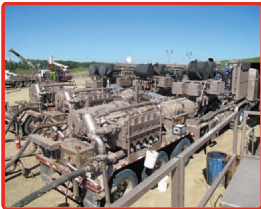
Trican fracturing operation with frac pumpers is shown. (Photo courtesy of Trican Well Service)
