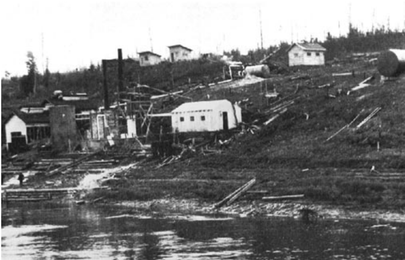
Early bitumen production in the 1930s near Fort McMurray. (Photo courtesy of Canadian Association of Petroleum Producers)
