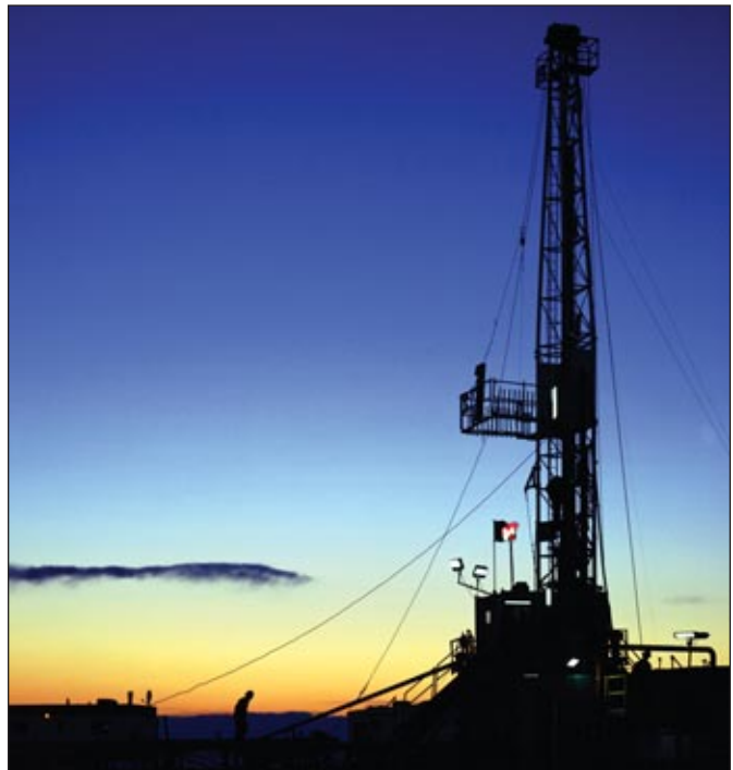
A rig at daybreak drills a coalbed methane well for MGV Energy Inc., a subsidiary of Quicksilver Resources. (Photo by Alberta Photo Co. courtesy of Quicksilver Resources)
