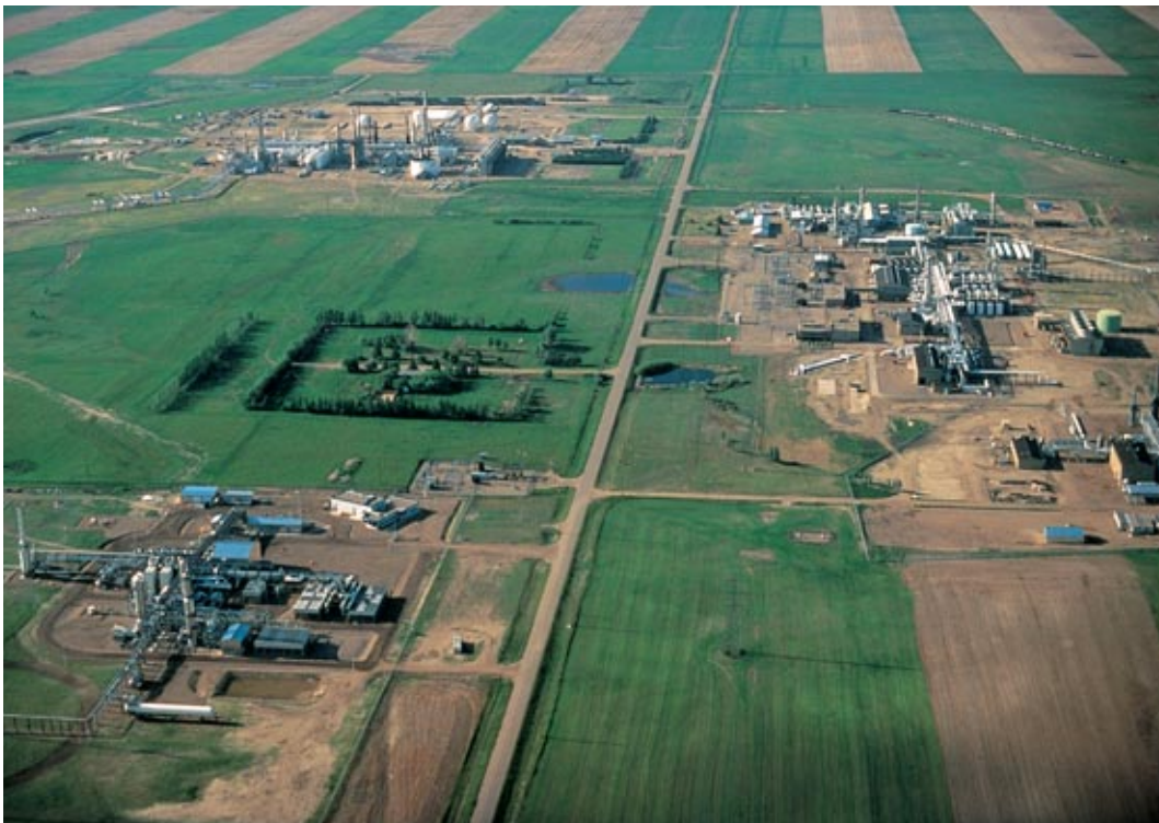
Five pipelines converge here at the Alberta border; one of the largest centers of gas compression in North America. (Photo by Lowell Georgia)
