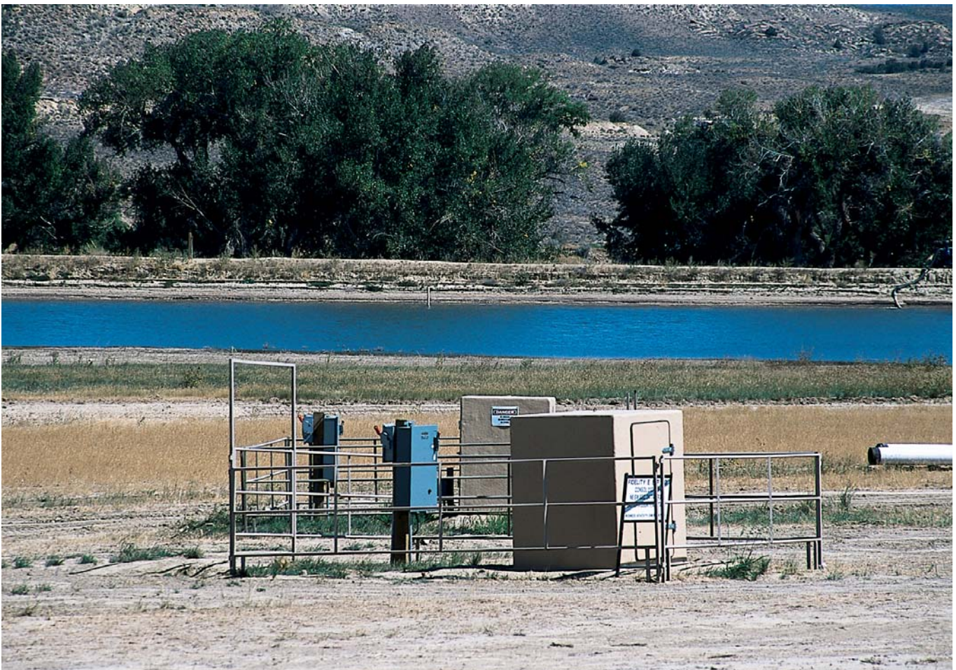
Surface impoundments are often used to contain the produced water from coalbed wells. (Photo by Lowell Georgia)
