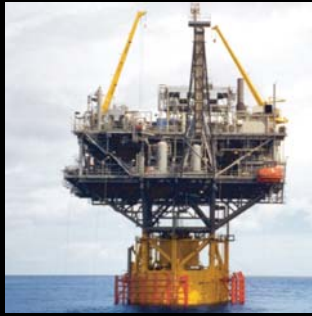
AGIP / ALLEGHENY FIELD 1999 Water depth 3,350ft. (1,021 m)
