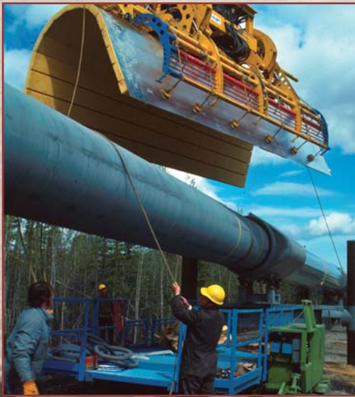
Workers oversee pipe installation on the Trans-Alaska oil pipeline.
