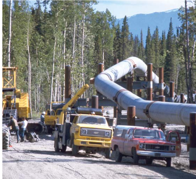
The pipeline above is shown being put on vertical support members.
