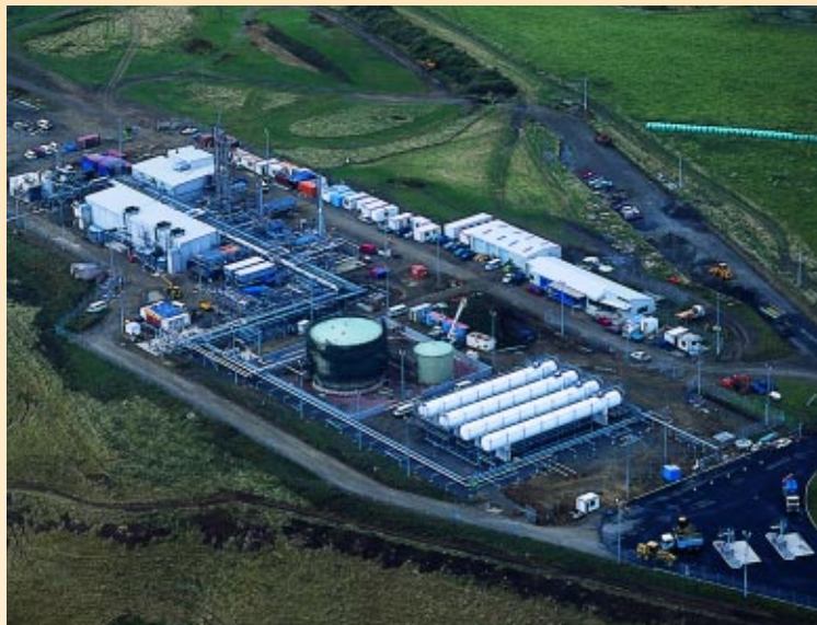
More mid-sized independents are finding reserves overseas to augment their U.S. activity. Here, Swift Energy's Rimu production station in New Zealand has capacity for 3,500 bbl of oil and 10 Mcfd of gas.
