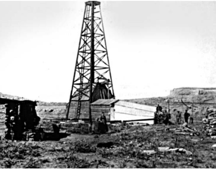
M.P. Shannon drilled the I Shannon in 1889 with the first standard drilling rig, a cable-tool unit, in the Salt Creek field area.
