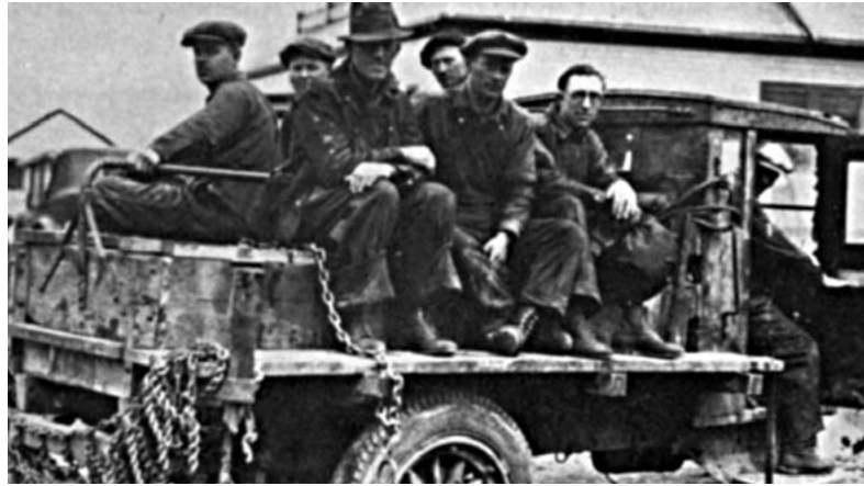
An early rig-building crew moved from site to site in Wyoming setting up and tearing down cable-tool drilling rigs.
