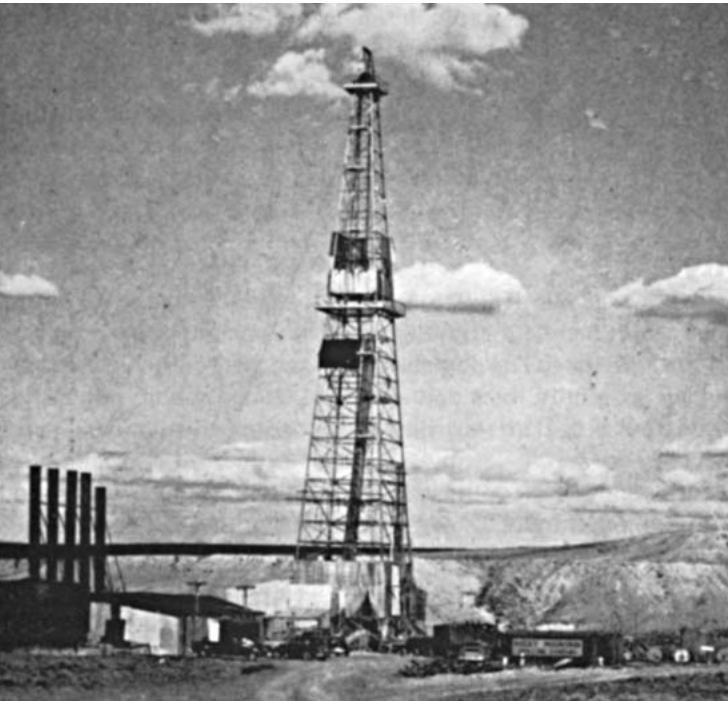
Mountain Fuel Supply (now Questar Corp.) drilled the deepest well in the Rockies when its Church Buttes discovery well went to 12,895ft. (Photo courtesy of Questar Corp.)
