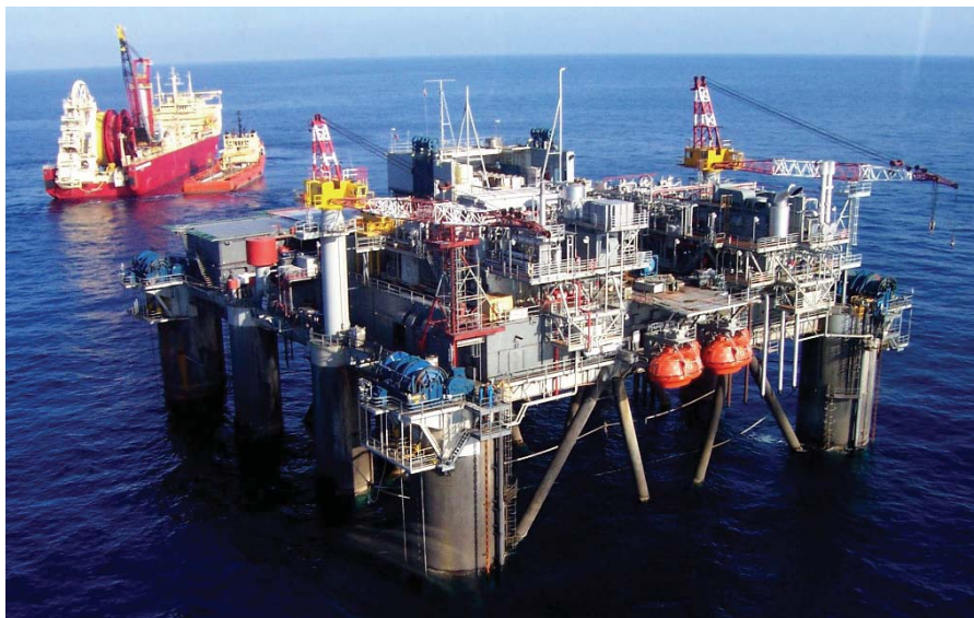
Phase II development is in progress at ATP's Mississippi Canyon 711. (Photo courtesy of ATP Oil & Gas Corp.)
