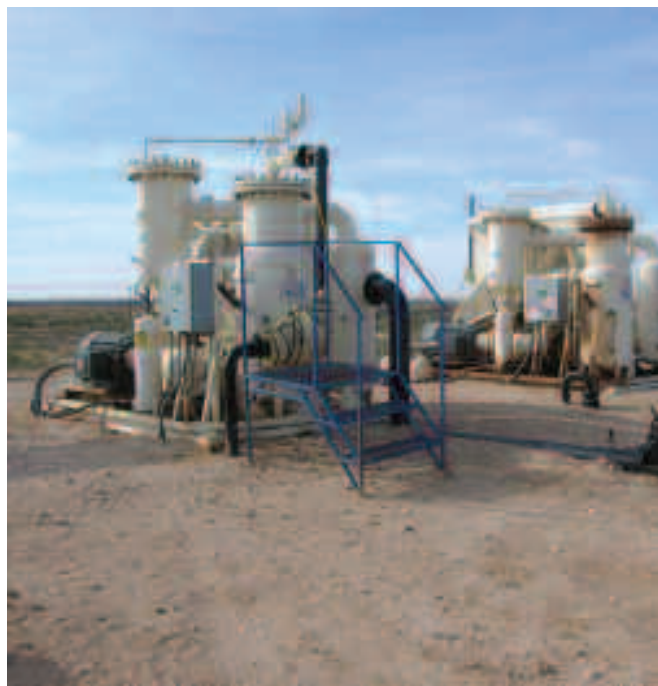
By early 2006, Stallion Energy had revamped most of the infrastructure.
