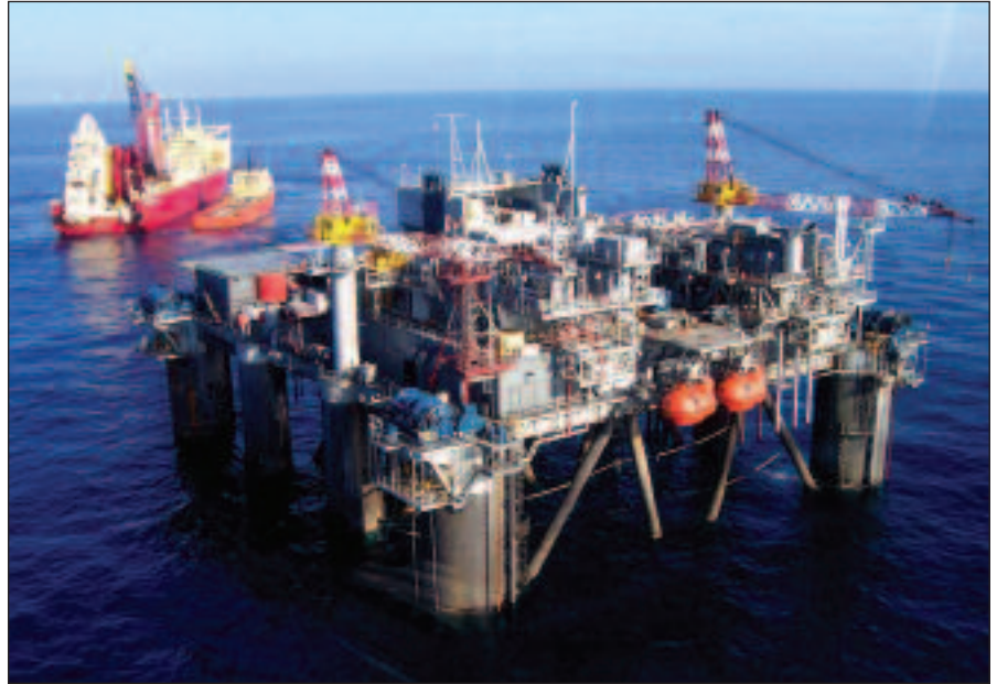
Phase II development is in progress at ATP's Mississippi Canyon 711.
