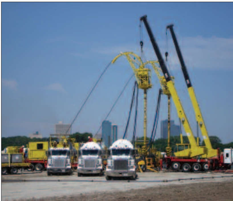
This Barnett Shale picture shows Parallel's simultaneous drilling frac plugs on two recently "simu-frac'd" wells utilizing coiled tubing units and downhole motors. Downtown Fort Worth, Texas, is shown in the background.
