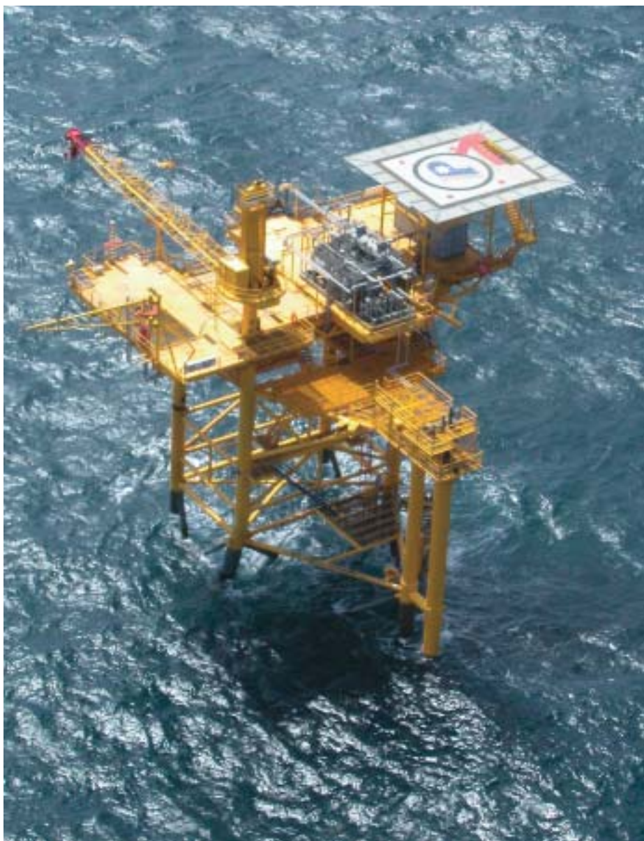
Petsec's Vermilion 258 platform in the Gulf of Mexico.
