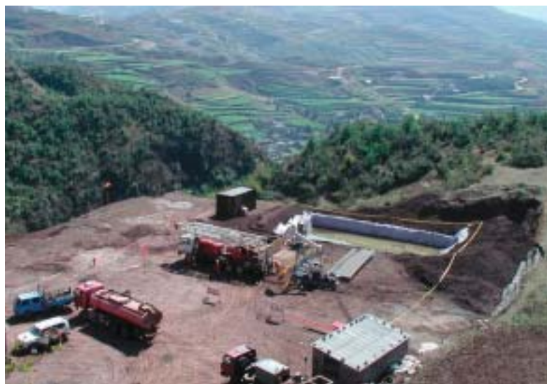
Far East Energy EH-01 well-test in Yunnan Province, China.
