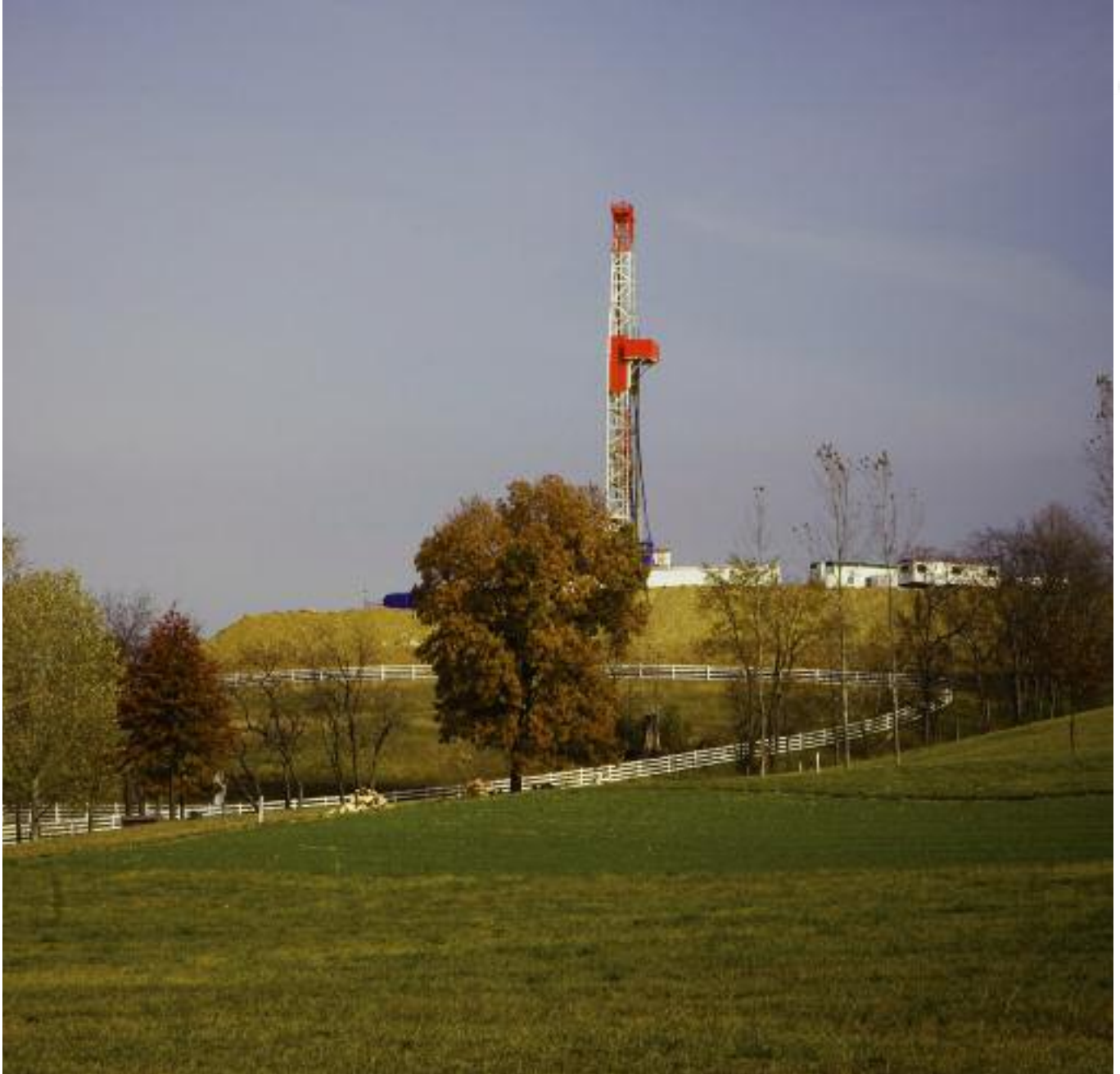
Range Resources Corp. has drilled nearly 100 wells in the Marcellus shale. (Photo courtesy Range Resources Corp.)
