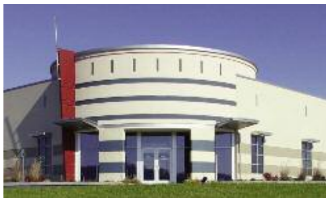
This is CNX Gas Corp.'s new Mountaineer headquarters in Pennsylvania. (Photos courtesy CNX gas)
