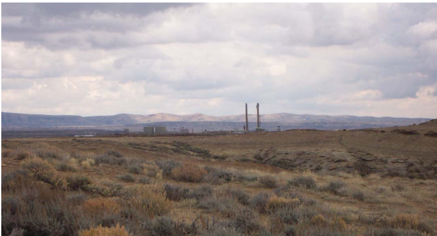
Distant view of Canyon Creek gas plant in the Vermillion Basin. (Photo courtesy of Questar E&P)
