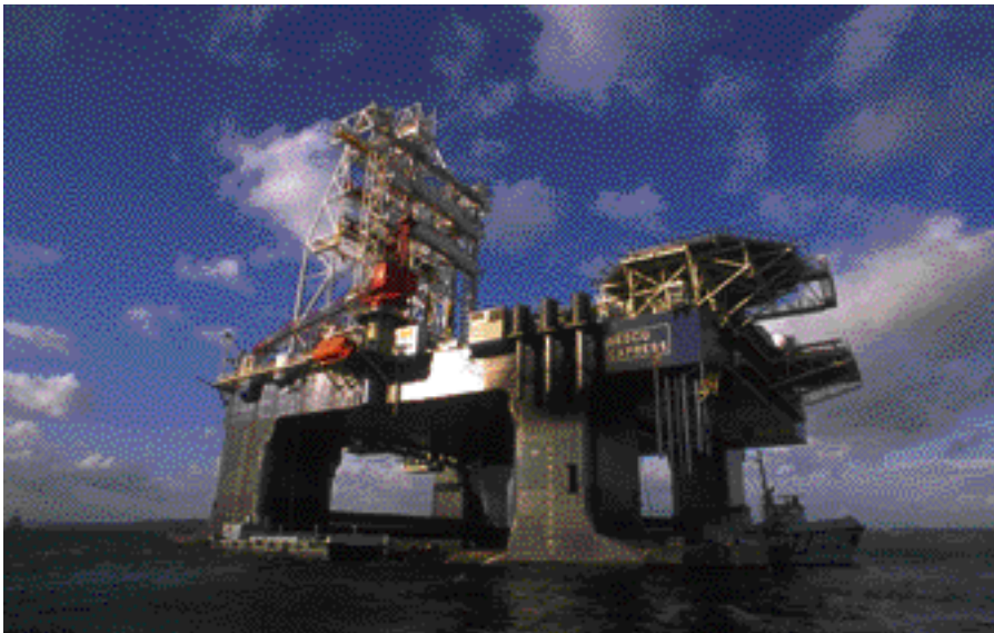
Transocean's Sedco Express features the Tri-Act derrick. The rig and two sister units— Sedco Energy and Cajun Express —feature penetration rates, streamlined logistics, extensive mechanization and parallel tubular handling operations that are supported by a transparent integrated well construction center.
