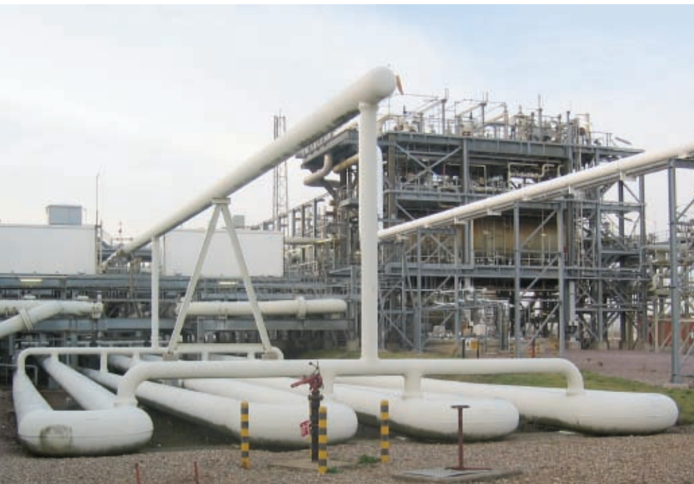
Above, a slug-catcher at Tullow Oil's gas terminal in Bacton. At right, Tullow Oil chief executive Aidan Heavey, who says there used to be a "big company" approach to the U.K. North Sea—usually expensive and slow—but that has been changing.
