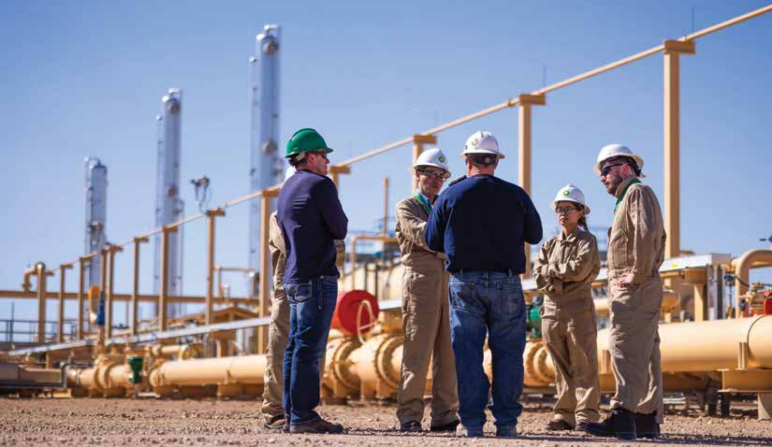
BP employees tour and discuss BPX's Grand Slam centralized processing facility in the Permian.
