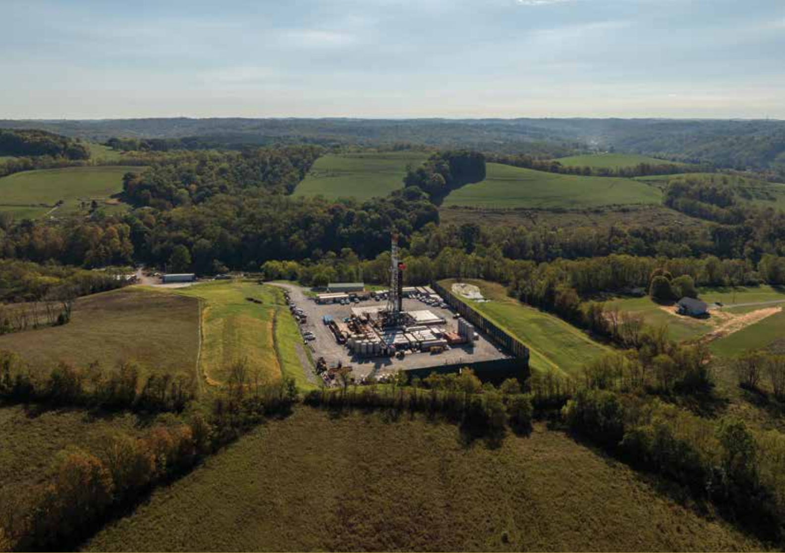
Drilling rig on location for Range Resources in southwestern Pennsylvania in October 2024.
